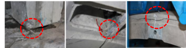
Cracks and damages of Rebar reinforced segment
